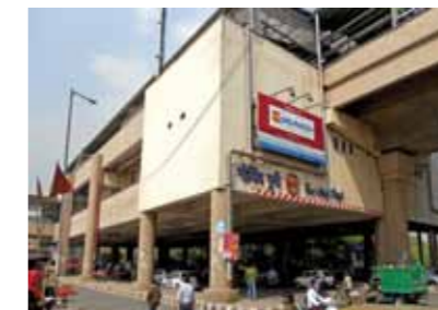
Govindpuri Metro Station
